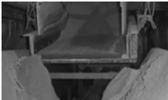
FMC Syntron vibratory pan feeder after TIVAR® 88 liner installation.
