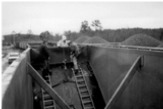
TIVAR® 88-2 end wall liner installation in progress.
